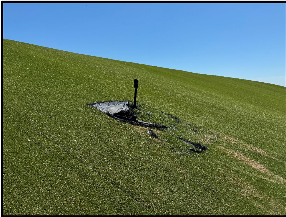
Photograph 2: Damaged closure turf around vent pipe near LCS-4.
