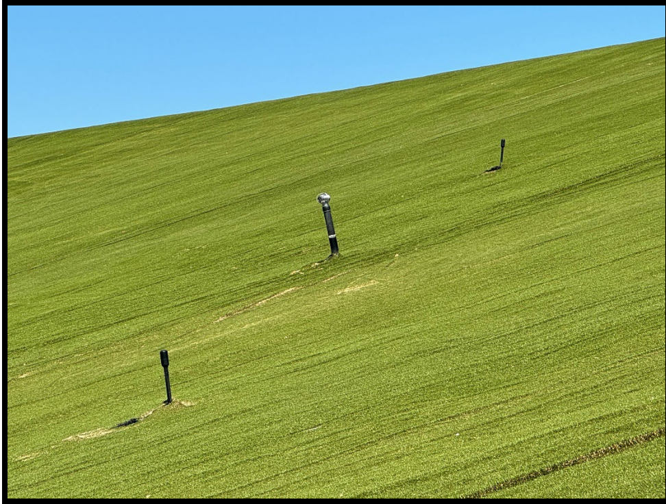
Photograph 1: Damaged closure turf around vent pipe near LCS-4.
